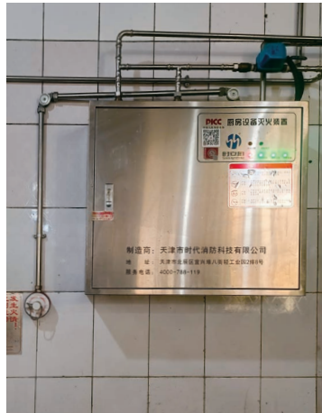
天津食品廠食堂自動滅火 及油煙淨化 Automatic fire extinguishing and grease purification for Tianjin food factory and its canteen
